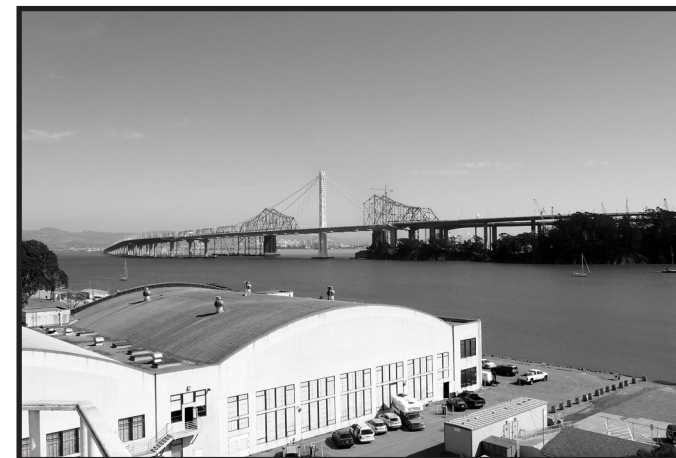
View from the outside of the Control Tower
